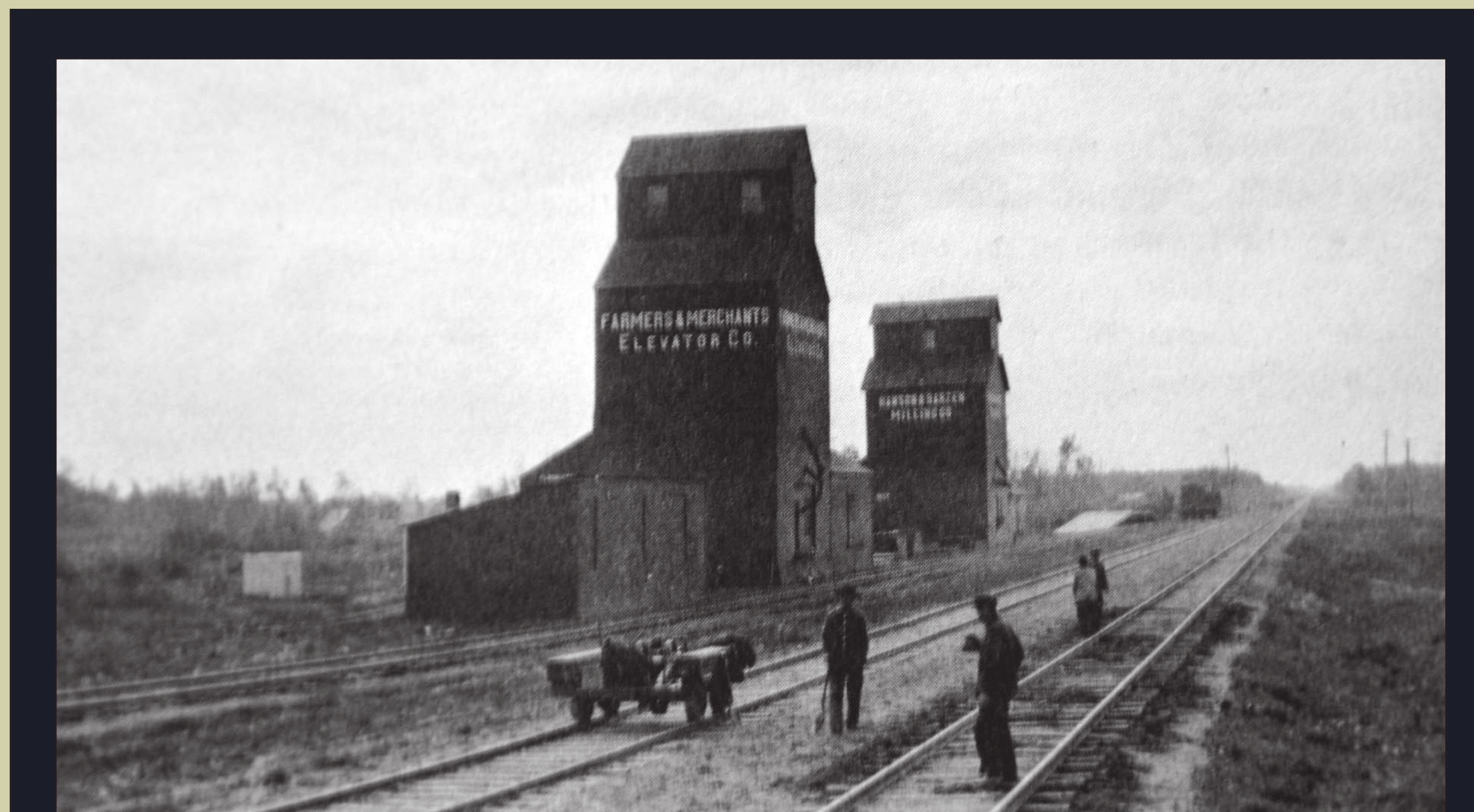
Looking south at the Farmers & Merchants and the Hanson & Barzen Elevators. Circa 1912.
