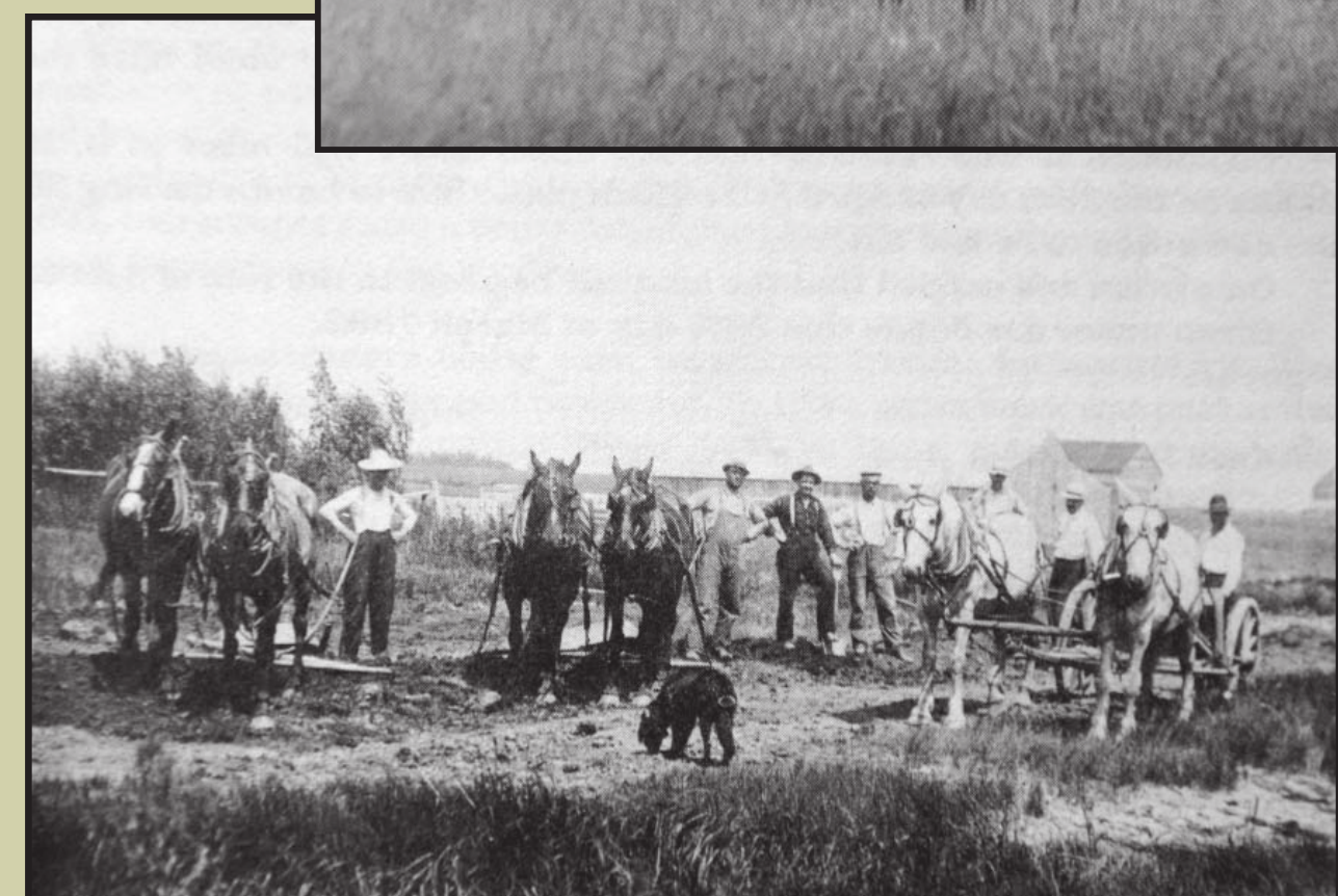
Above: A typical mode of transportation in the 1800s. Below: A road building crew in New Folden Township. Circa 1890s.
