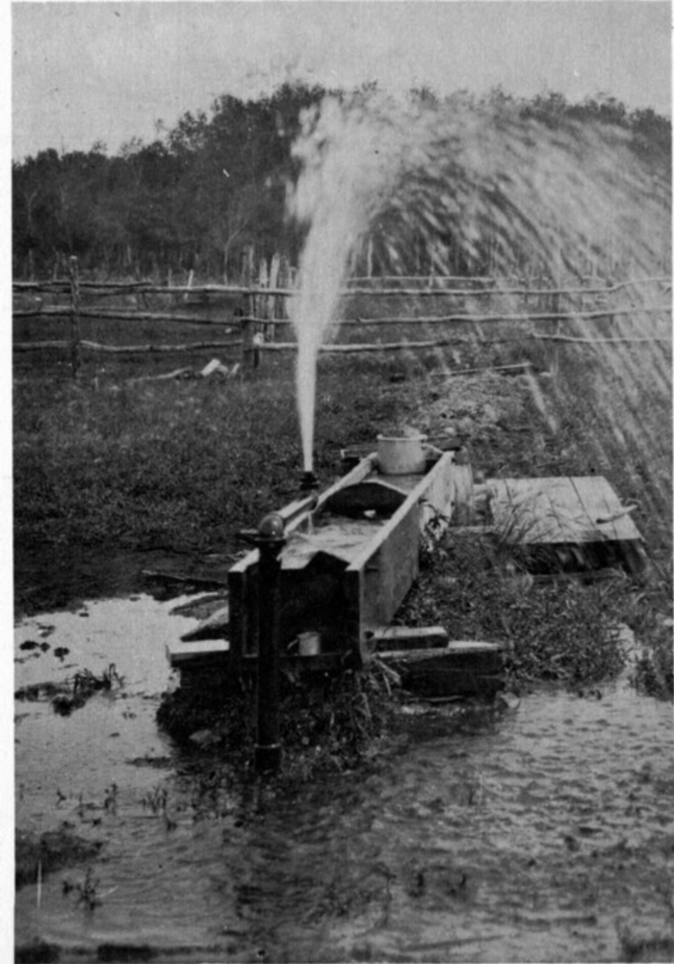
A powerful flowing well drilled in 1908 by Ole Ihle on the John Knutson homestead, spouting water 20 feet above ground level. The S.E. ¼ Sec. 22 Marsh Grove Twp.
