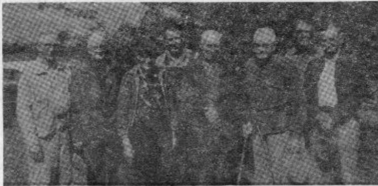
1958 Newfolden Central Telephone Board
